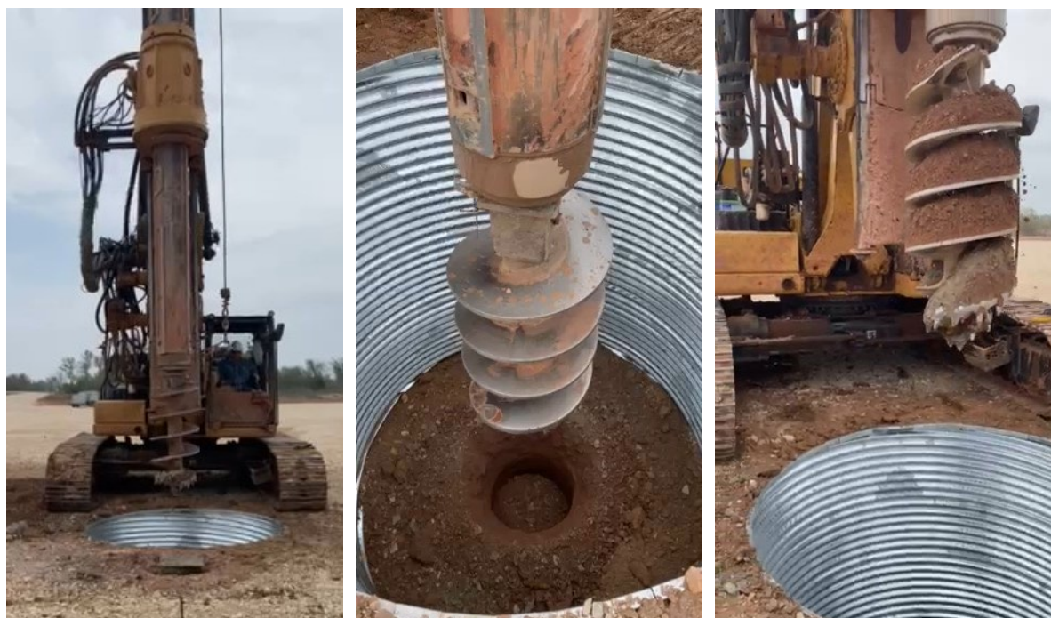
Figure 1. Drilling of the Jewell Well conductor casing hole using a specialised auger drill
